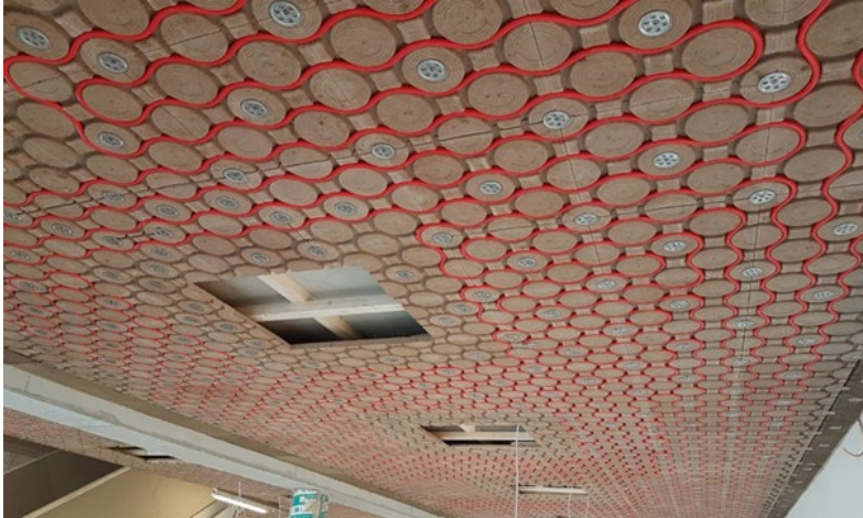
Fixing to substructure formwork with various ceiling outlets
