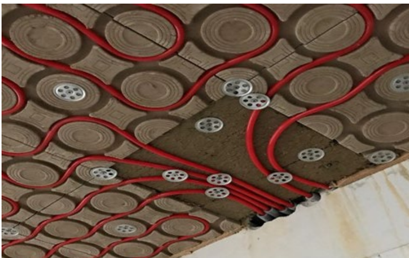
Connection surface with 13mm clay connection plate as plaster base
