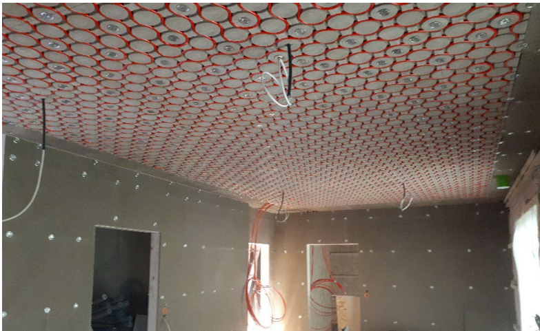
Full-surface ceiling covering with high-performance clay modules and clay neutral panels
